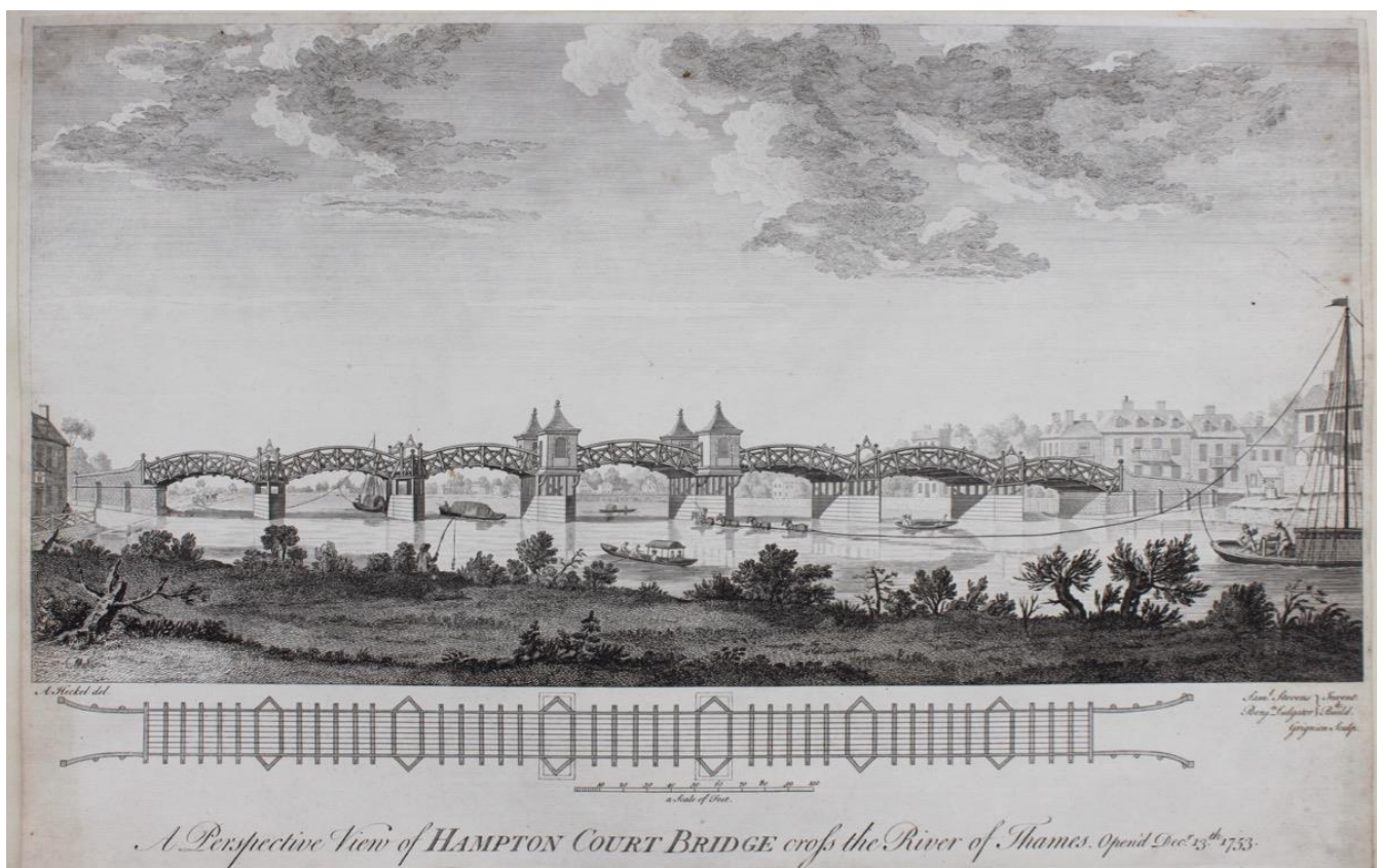
17. HECKEL, A[ugustin] A Perspective View of Hampton Court Bridge Cross the River Thames. Open'd Decr. 13th 1753. Charles Grignon, c. 1765? Engraved print, c. 320 x 550 mm. A fine example. This, the first bridge on this site, was completed in 1753, but replaced in 1778. Augustin Heckel was born in Austria but came to England as a young man where he worked as a watch case engraver and painter; he died in Richmond in 1770. £350
